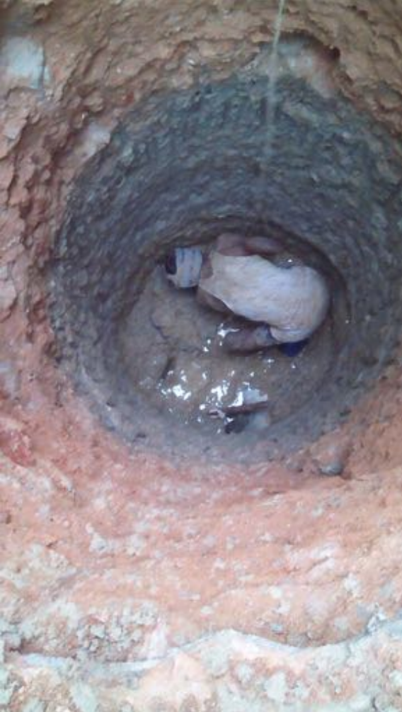
The soil is excavated to the required depth
