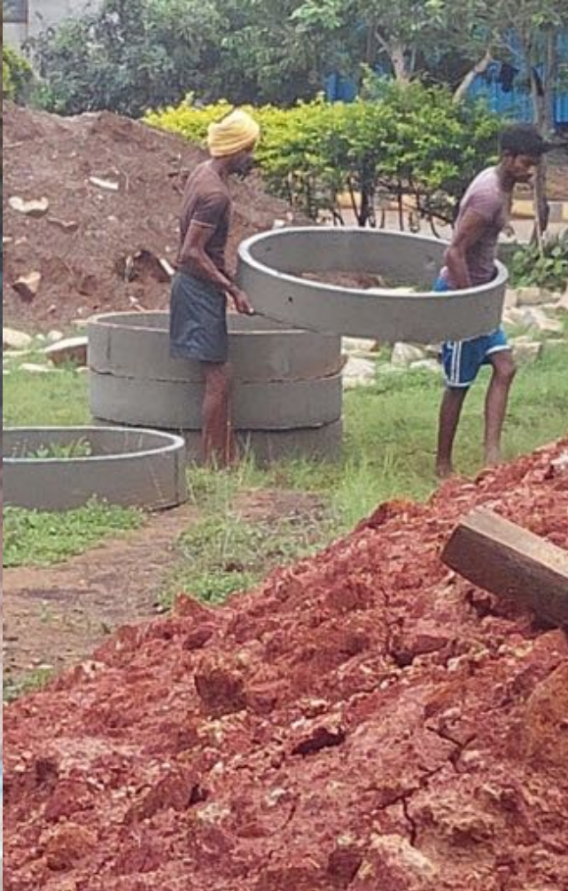
Concrete rings are lowered in one by one into the well
