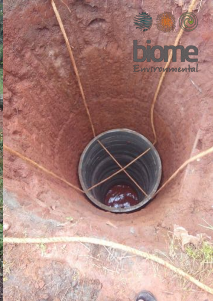
This reinforces the well structure
