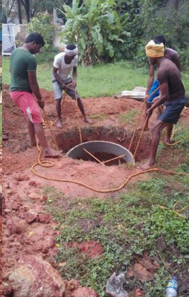
Aggregate or jelly stones line the gaps between the rings
