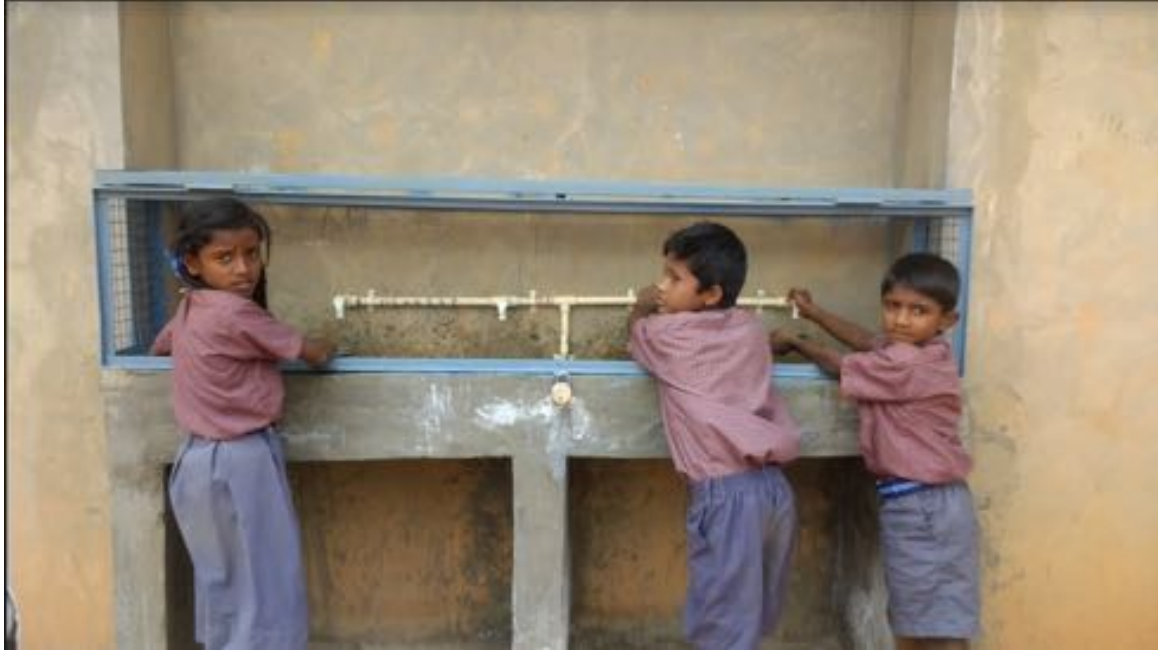
Hand wash was built with a mesh around to prevent incidences of vandalism
